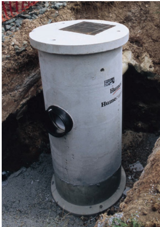
Left: HumeCeptor® STC2 with extended bypass chamber and Kor'N'Seal boots.
