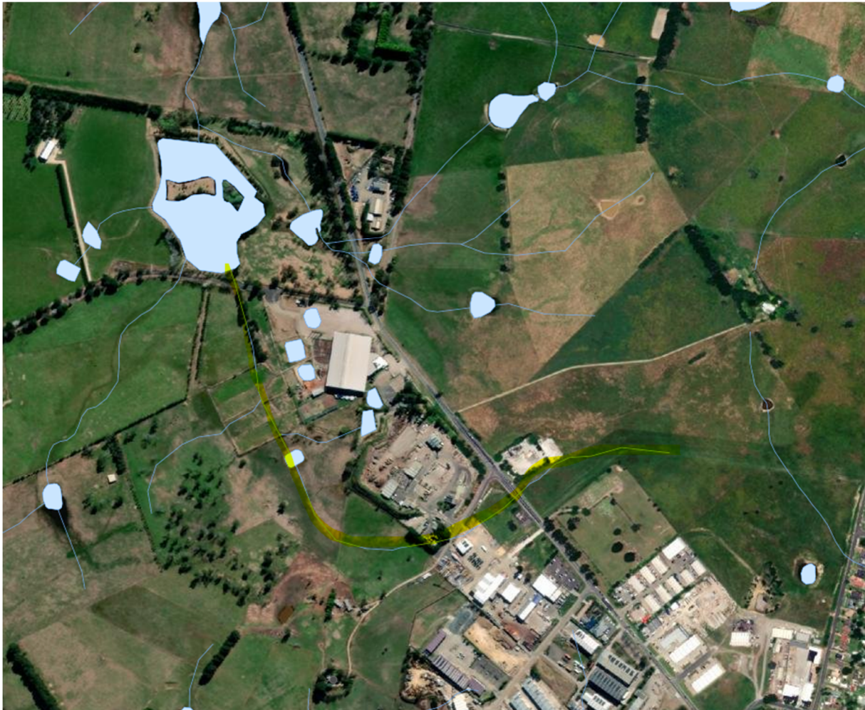
Figure 3.1: Identification of existing northern watercourse impacting the development site (NSW Water Management Regulation 2018)
