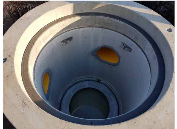
Above: Base, shaft, and surround installed
