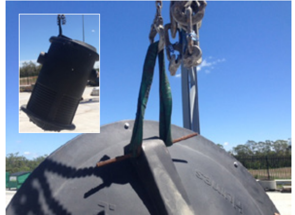
Figure 3 – Lifting using a bar and soft sling
